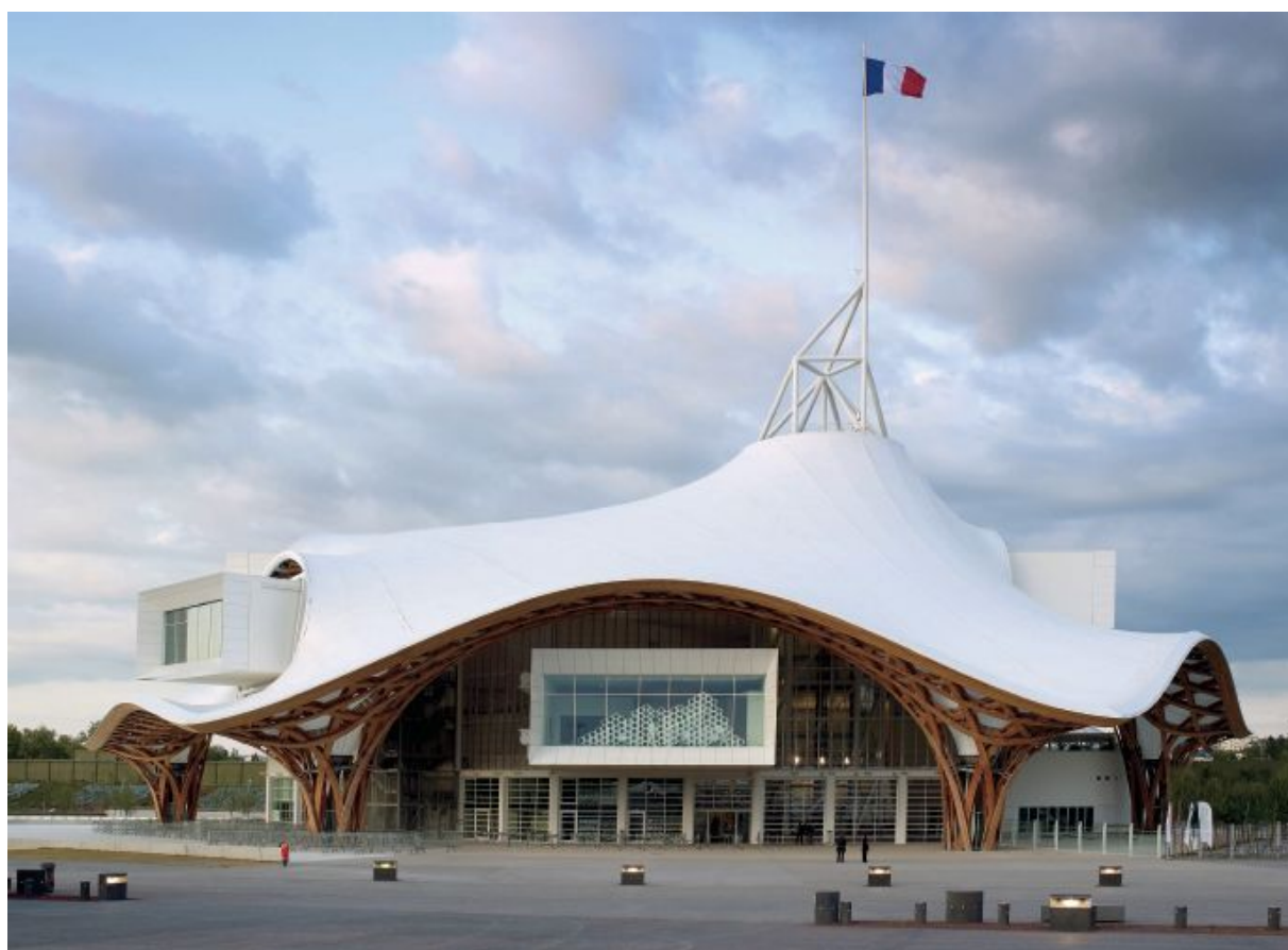
13.32 Shigeru Ban. Centre Pompidou-Metz, Metz, France. 2010. flashover/Alamy Stock Photo
