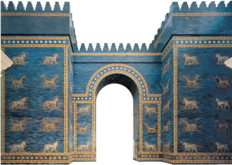
14.9 Ishtar Gate (restored), from Babylon. ca. 575 B.C.E. Glazed brick, height 48' 9".
