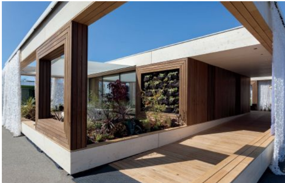
13.39 Team Austria. LISI House, Irvine, California. October 10–13, 2013. Jason Flakes/U.S. Department of Energy Solar Decathlon
