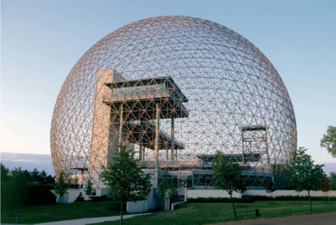
13.30 R. Buckminster Fuller. U.S. Pavilion, Expo 67, Montreal. 1967. Geodesic dome, diameter 250'.
