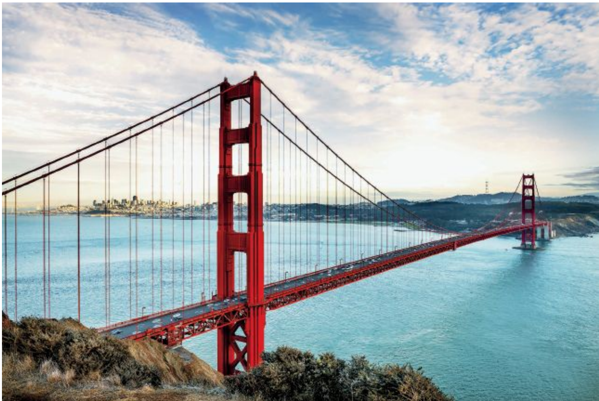
13.26 Golden Gate Bridge, San Francisco. 1937. Joseph B. Strauss, chief engineer; O. H. Ammann, Charles Derleth, Jr., and Leon S. Moisseiff, consulting engineers; Irving F. Morrow, consulting architect.
