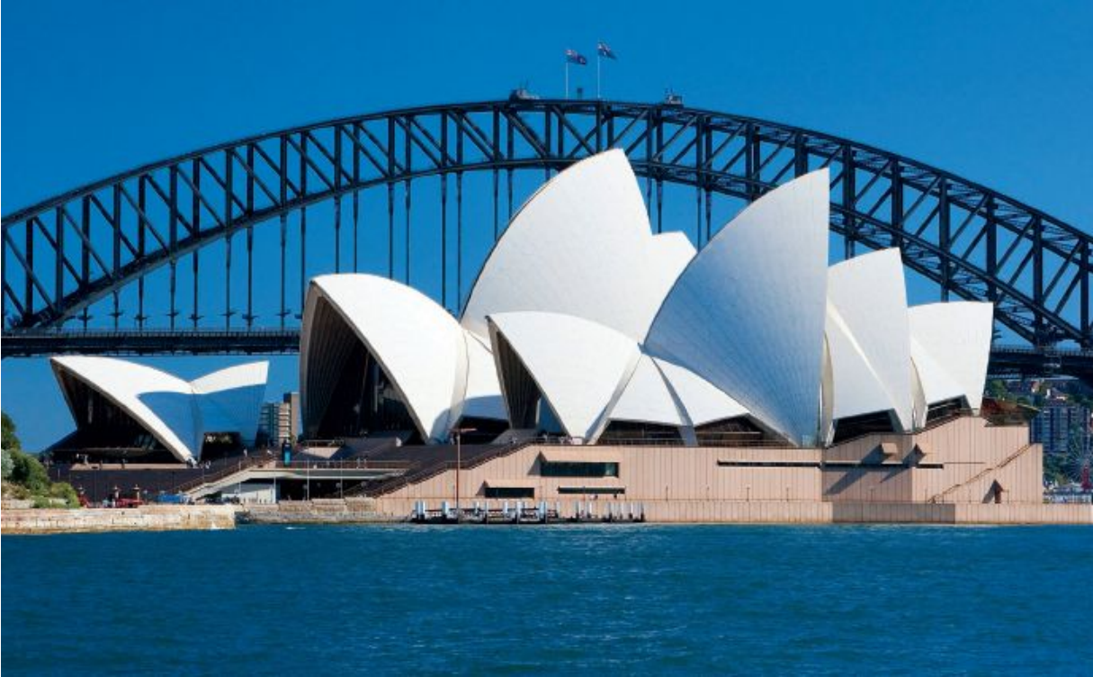
13.28 Jørn Utzon. Sydney Opera House, Australia. 1959–72. Reinforced concrete, height of highest shell 200'.
