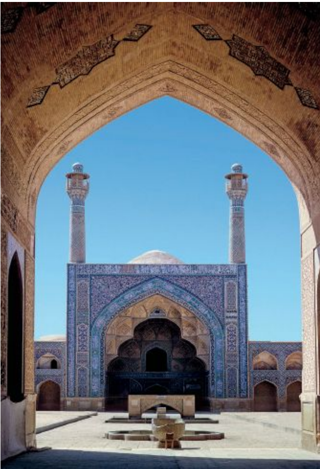
18.4 Qibla iwān , Friday Mosque, Isfahan. Rebuilt after 1121–22 (with later work).
