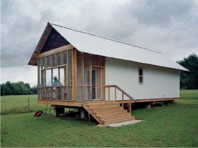
13.36 Rural Studio. 20Kv08 (Dave's Home), Newbern, Alabama. 2009.
