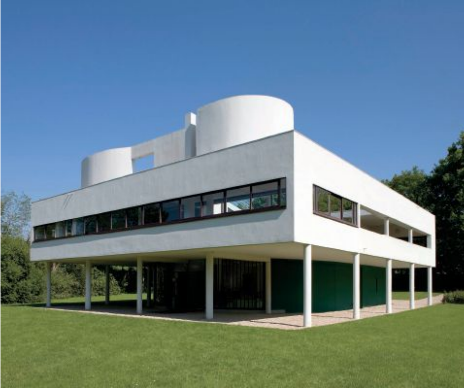
5.25 Le Corbusier. Villa Savoye (Villa les Heures Claires), view from northwest. 1928–31.
