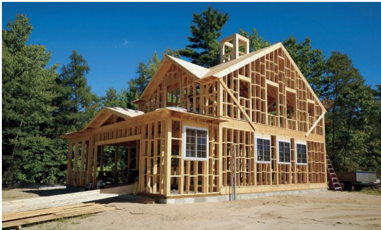
13.23 Balloon-frame house under construction.
