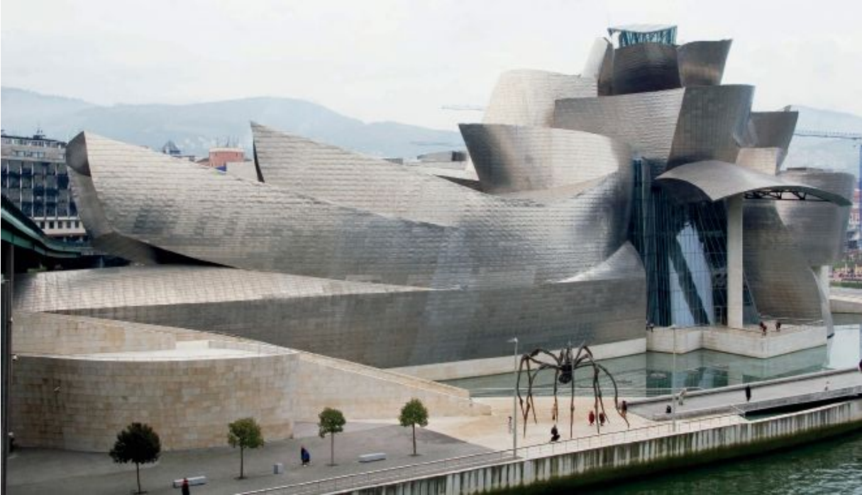
13.31 Frank Gehry. Guggenheim Museum Bilbao, Spain. 1997.
