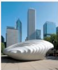
13.33 Hadid, Burnham Pavilion
