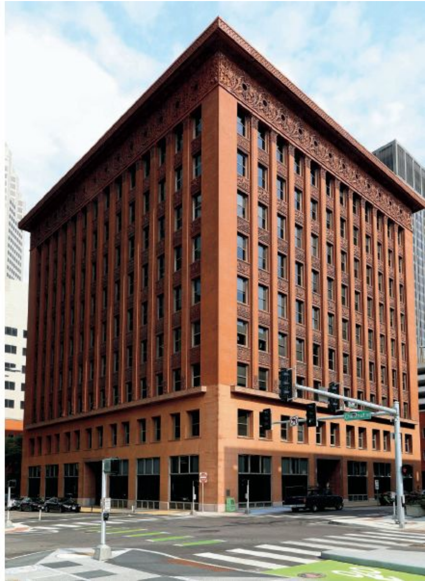
13.24 Louis Sullivan. Wainwright Building, St. Louis. 1890–91.
