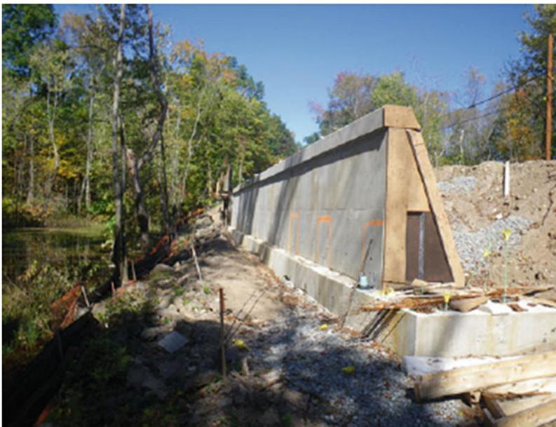
**Fig. 8.4** Cantilever wall construction
