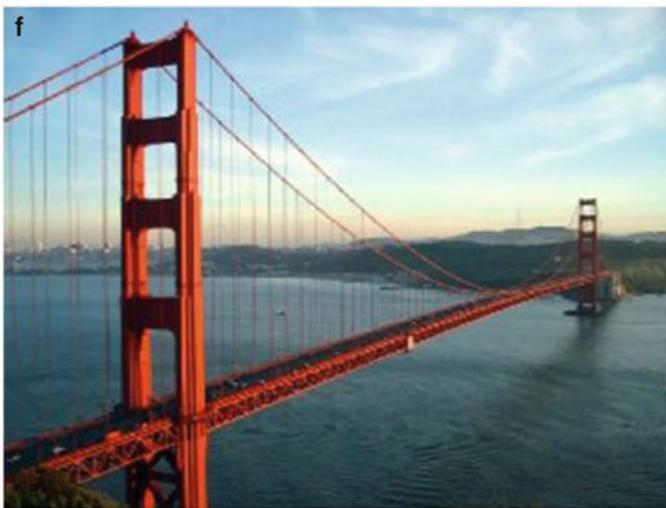
Cable-girder system (suspension bridge)
