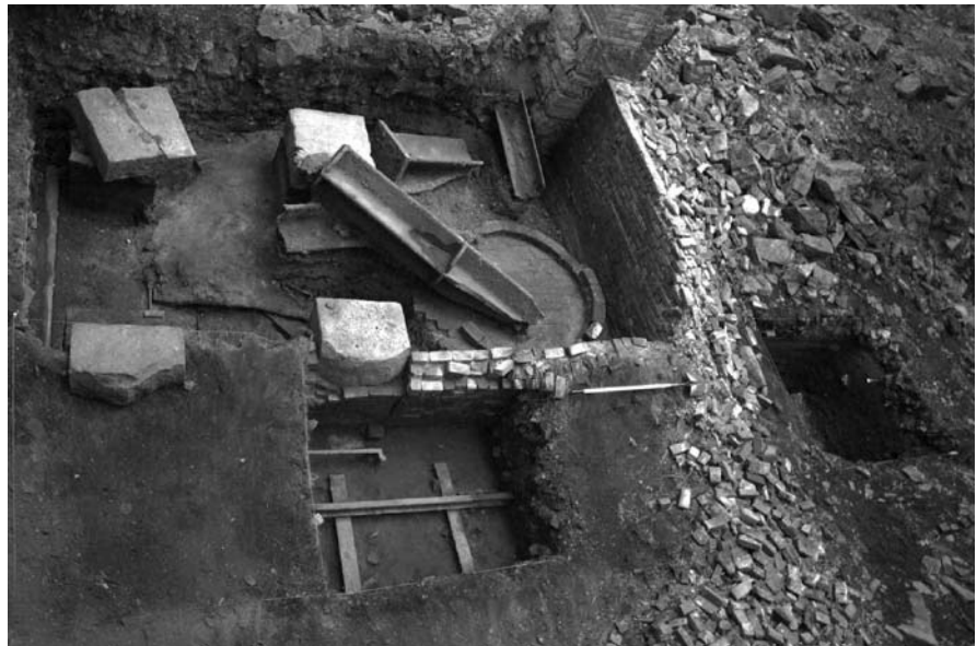
Fig. 4 Excavated ironworking cupola base, West Point Foundry, Cold Spring, New York (photograph by Michigan Technological University staff)
