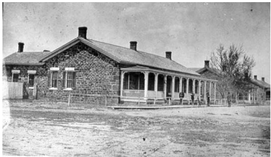
Fig. 1 The officers' quarters at Fort Larned, Kansas, exemplify the higher status that officers of the frontier Army enjoyed (Fort Larned National Historic Site photograph)
