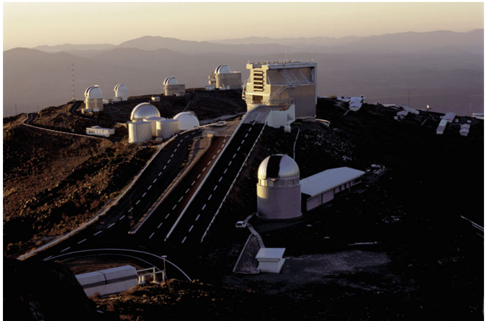
Fig. 1.36 The La Silla Observatory of ESO in Chile. On the peak in the middle, one can see the New Technology Telescope (NTT), a 3.5-m prototype of the VLT. The silvery shining dome to its left is the MPG/ESO 2.2-m telescope whose Wide Field Imager, a 8096^2 pixel camera with a 0.5^\circ field-of-view, has been a very competitive instrument in the past decade. The picture was taken from the location of the 3.6-m telescope, the largest one on La Silla. Credit: European Southern Observatory
