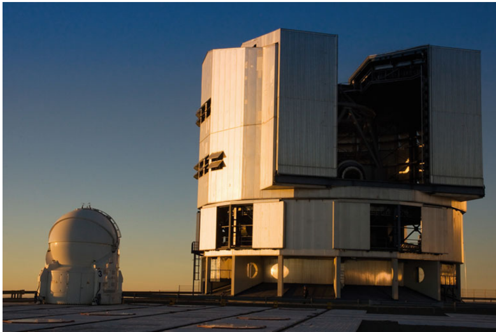
Fig. 1.42 One of the four Unit Telescopes of the VLT on the right, together with one of the auxiliary telescopes at the left. These auxiliary telescopes can be moved to allow for variable baseline configurations
