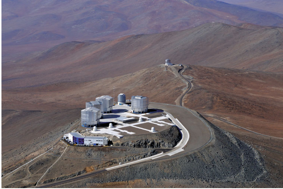
Fig. 1.39 The Paranal observatory after completion. The four large domes host one of the VLTs each. The smaller dome, seen to the left of the rightmost VLT, hosts the VLT Survey Telescope (VST), a dedicated 2.6 m telescope equipped with the wide-field optical camera Omega-CAM. The four much smaller domes host 1.5 m auxiliary telescopes, which are used in combination with the VLTs for optical interferometry. In the background, the VISTA (Visible and Infrared Survey Telescope
