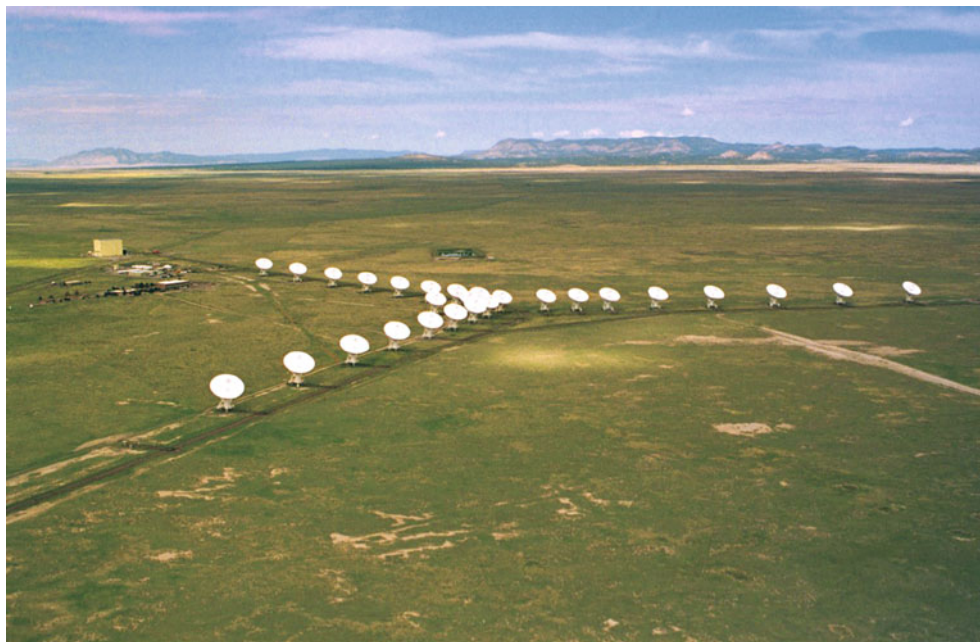
Fig. 1.26 The Very Large Array (VLA) in New Mexico consists of 27 antennas with a diameter of 25 m each that can be moved on rails. It is used in four different configurations that vary in the separation of the telescopes; switching configurations takes about 2 weeks. Credit: NRAO/AUI
