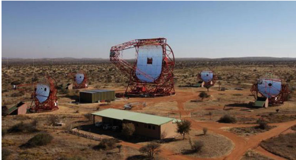
Fig. 1.50 The four 13 m-diameter telescopes, and the new 28-m telescope of the High Energy Stereoscopic System (H.E.S.S.) in Namibia, in South-West Africa. The optical quality of these mirrors is much lower than that of other optical telescopes. The angular resolution of the telescopes needs not to be better than a few arcminutes, as
