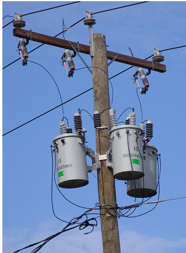
Figure 15.21 Transformers are used to step down the high voltages in transmission lines to the 110 to 220 V used in homes. (credit: modification of work by “Fortyseven”/Flickr)
