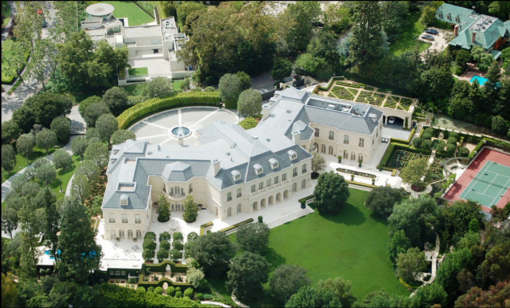
FIGURE 9.1 This house, formerly owned by the famous television producer, Aaron Spelling, sold in 2019 for $119 million, which set the record for the highest individual home sale in California history. It is the largest private home in Los Angeles, and is considered one of the most extravagant homes in the United States. (Credit: Atwater Village Newbie/flickr)
